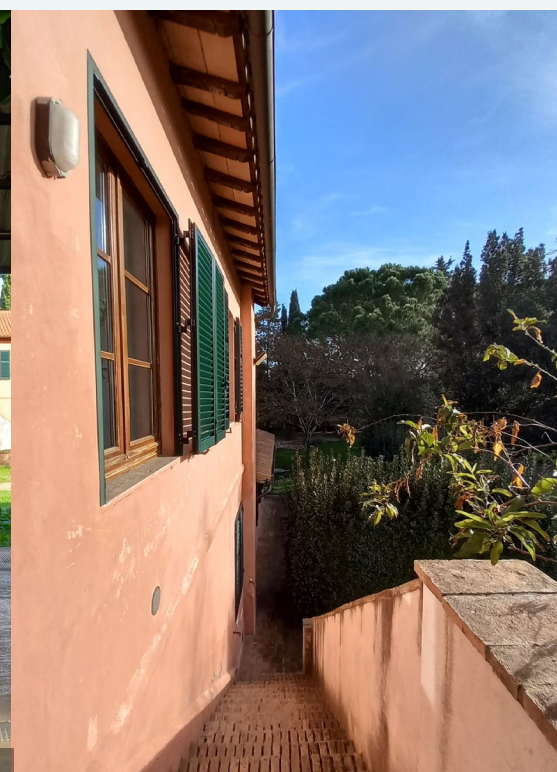
I Roggiati external stairs (photo by Lucia Tacconi and Jacopo Goracci)
